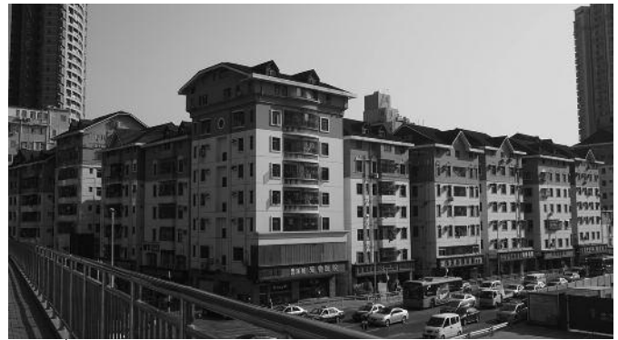
Photo 4 – Standardised building appearance.
